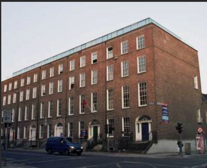
Work is ongoing at 80 – 84 O'Connell St. No.'s 80 and 81 have been completed with work to the remainder of the former County Council Offices due for completion in Spring 2009. The project involved the restoration and refurbishment of the existing Georgian buildings with their historical subdivision being reinstated and a new pristine glass roof extension to replace the double pitch roof which had been replaced in the 1970's with a flat roof.
